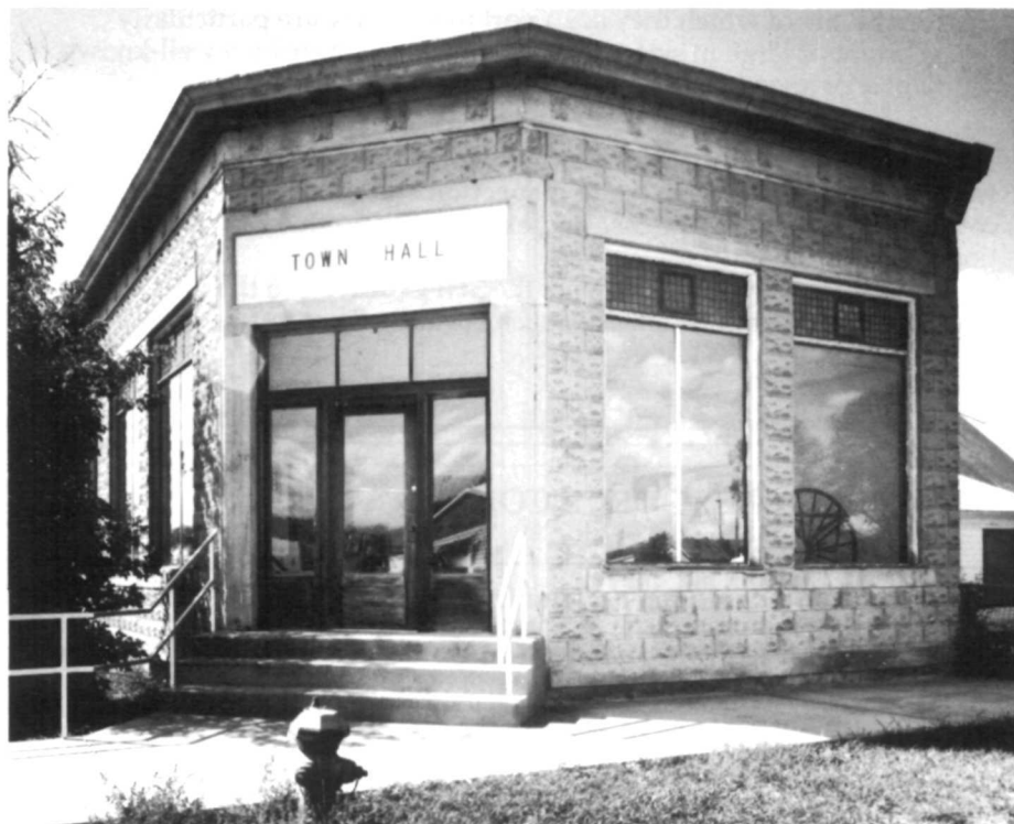
Functions and uses often change. Built as the Stockgrowers Bank in 1916, this building in Carbon County, Wyoming, became the Dixon Town Hall in 1975. By serving the region's farmers and ranchers from 1916 to 1923, the bank played an important role in fostering the frontier town's development. (Richard Collier)
