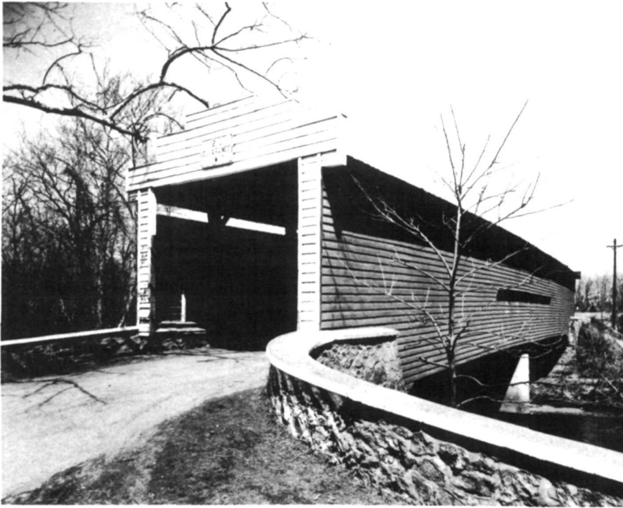
Hall's Bridge spanning French Creek, built about 1850 and 116 feet in length, is a surviving example of the Burr-truss design, which, invented in 1806, was a major advance in American bridge design. Over one hundred bridges of this type were built in Chester County, Pennsylvania, between 1812 and 1885. Hall's Bridge is one of the few remaining examples.
